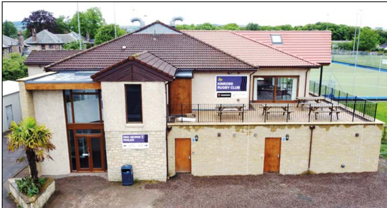
KGV Muirs Pavilion southern aspect showing new entrance atrium and terrace
